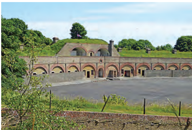
Central Haxo casemates with shifting lobby between, WWII blast walls evident within. Tunnel through to central caponier below. Photo Bob Clary
